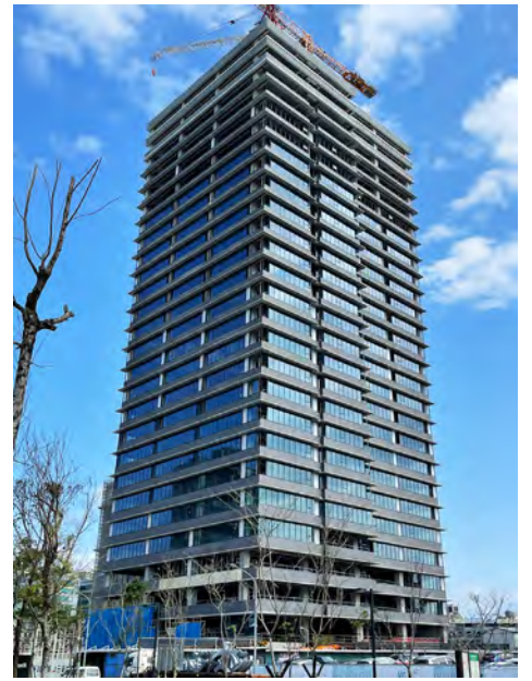
Fig. 3: A 27-story New RCS building in Nangang, Taipei, nearing completion.
