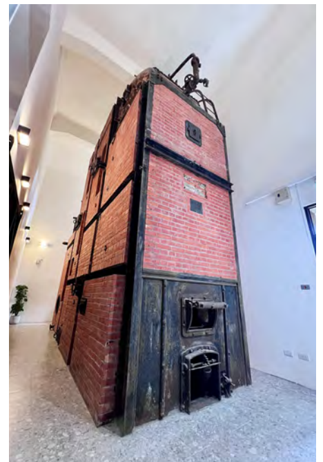
The boiler's 62 cm thick, red brick walls and 42 by 37 cm front gate.
