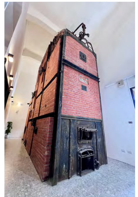
The boiler's 62 cm thick, red brick walls and 42 by 37 cm front gate.
