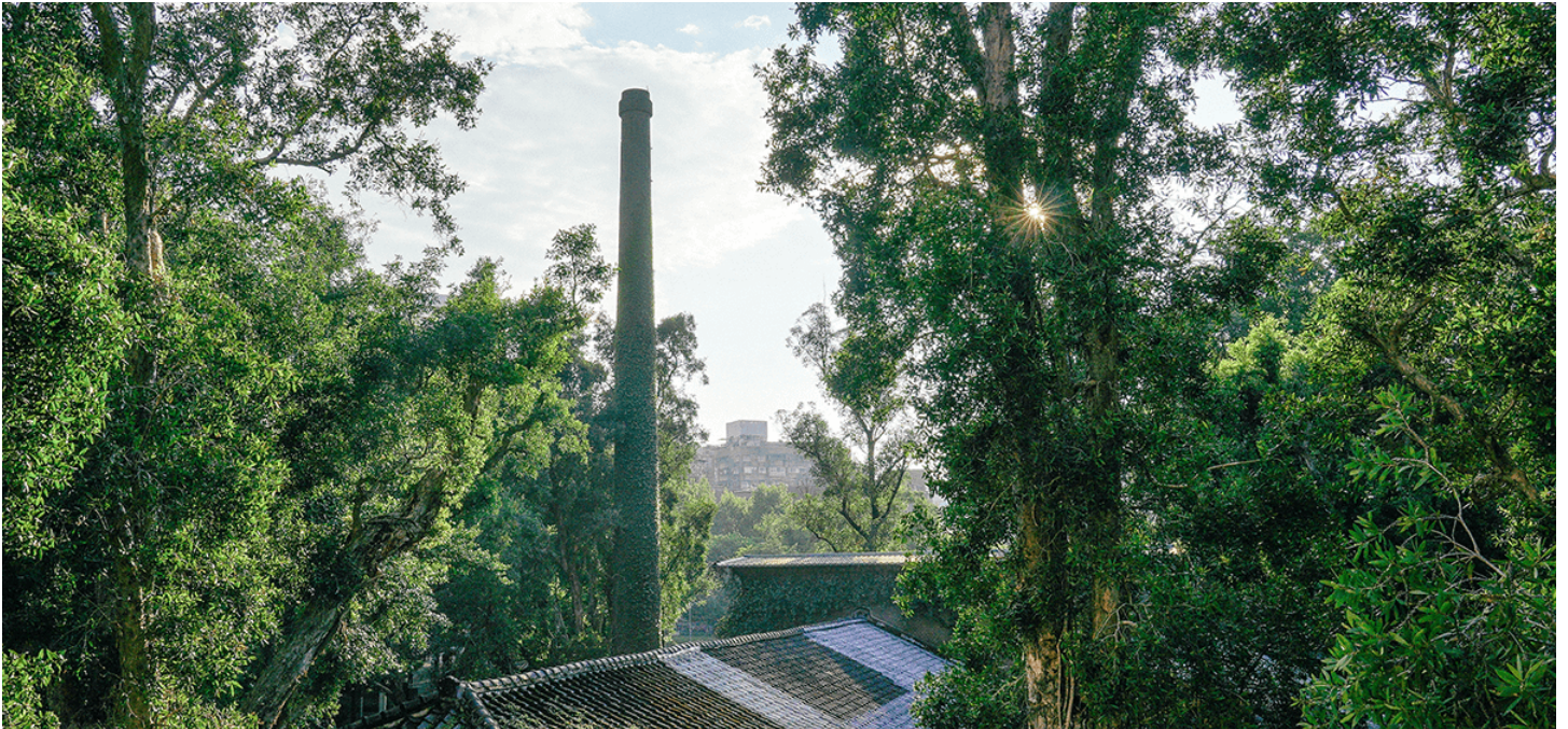
Completed on March 19, 1931, the chimney of the boiler room is nearly 20m in height and 6.188m in diameter.
