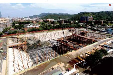
The construction team has created the hospital's subterranean levels through an approach called island excavation.
