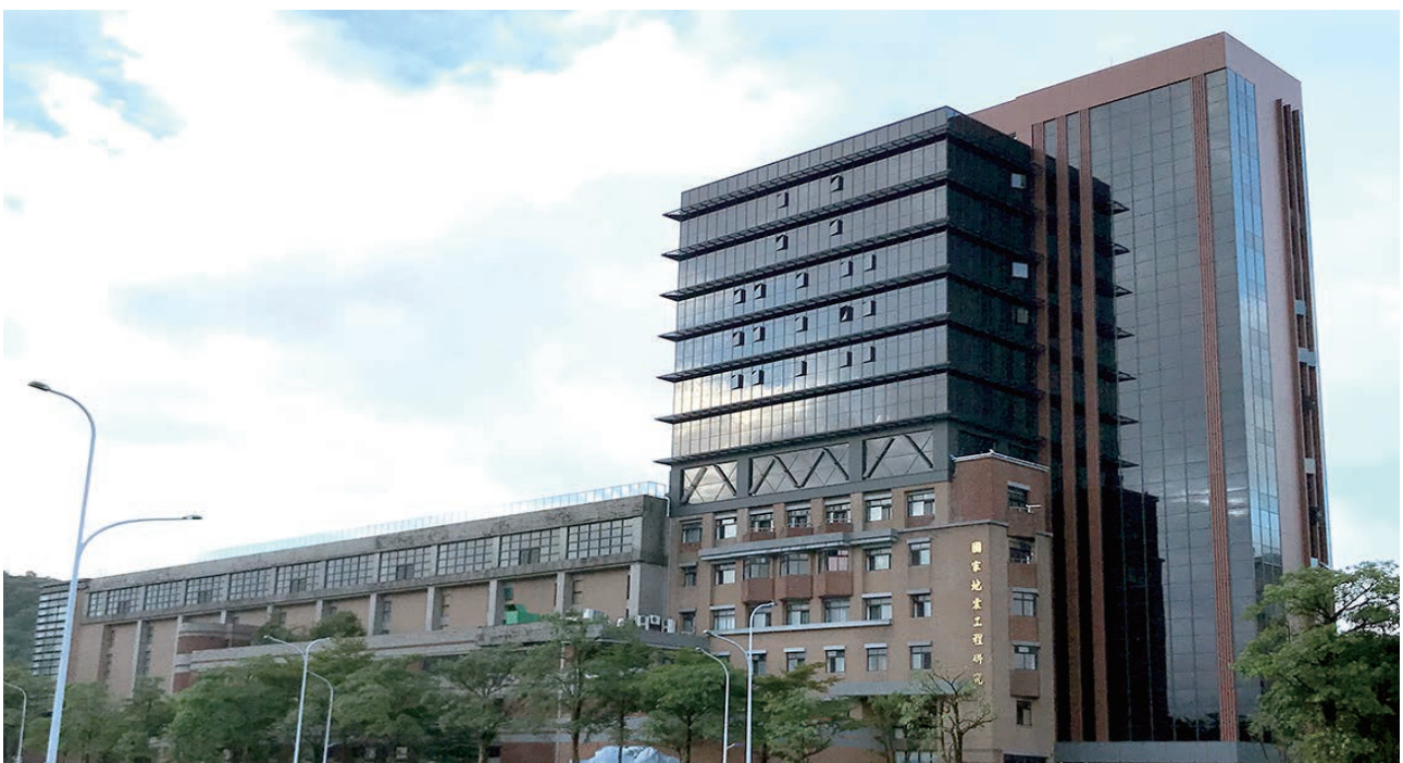
The extension of the NCREE building is an important benchmark for all smart earthquake-resistant buildings in Taiwan.
