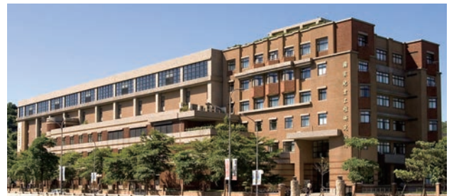
Photo prior to the extension shows that the project had to tackle the challenge of combining structures from different eras by connecting very different materials.
